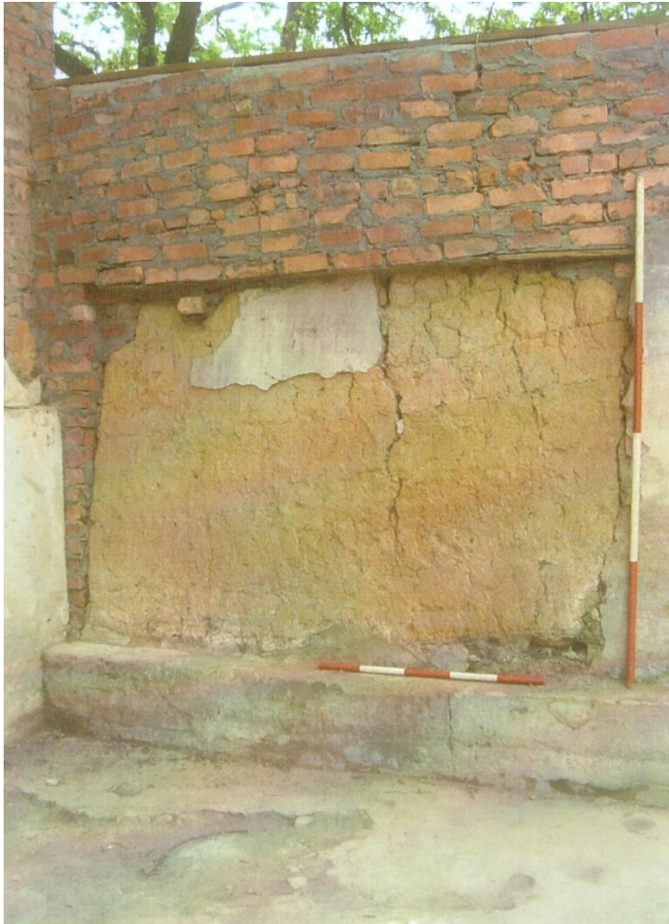
The oldest piece of wall on the farm, which dates to c1685-1700, was constructed with layers of compacted clay. This wall was covered in fresh plaster during the renovation, and is preserved in position.
