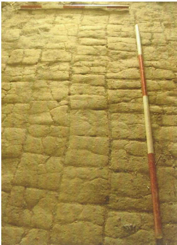
The tiled clay blocks forming the “brandsolder” on the ceiling, as fire proofing for the house below.
