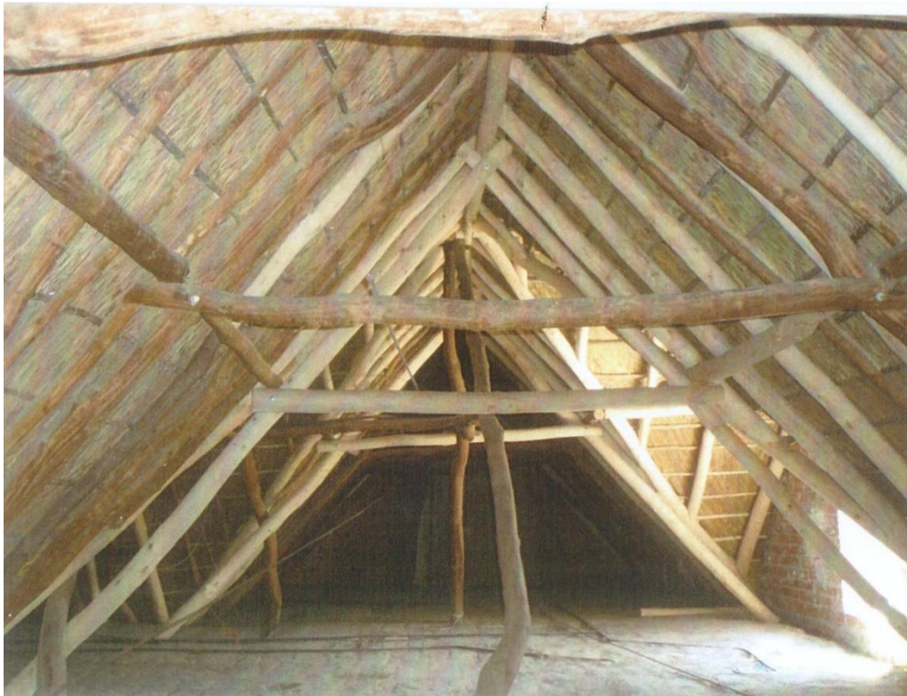
Original roof timbers have been conserved.
