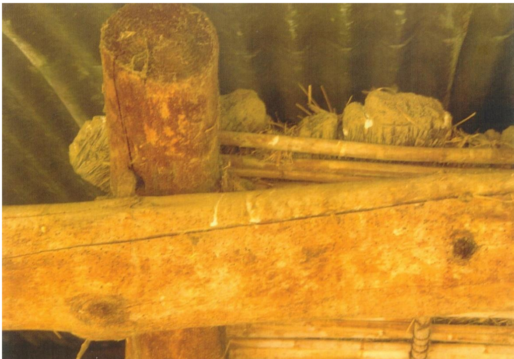
The original ceiling build up was still in place during the restoration. Note the reed ceiling, cross-reed tied with twine, the straw layer, and the clay "brandsolder" layer on top.
