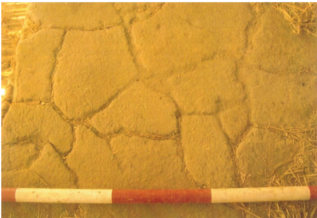
Clay “brandsolder” (fire-proofing layer) in the loft of “The Chapel”
