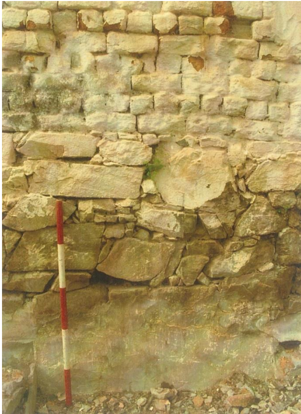
Foundation walling of Hornfels stone, with soft clay brick walls above
